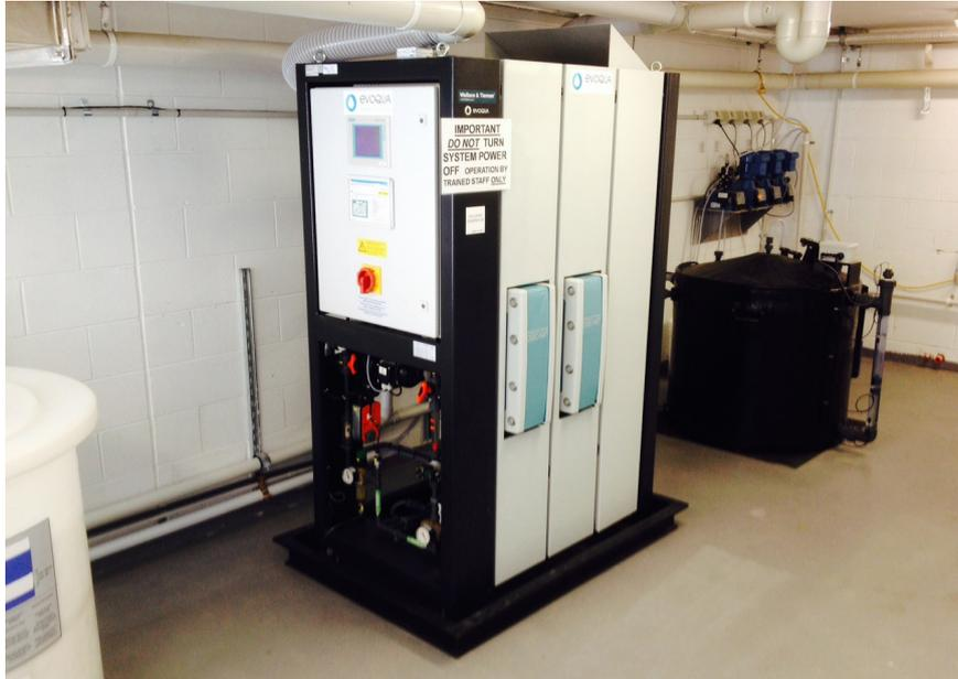
The Wallace & Tiernan OSEC-NXT 60 kg/day on-site chlorine generation system in use at MUR Holsworthy Army Base and the OSEC-NXT 24kg/Day system installed on the new Manly Aquatic Centre's indoor pools in Sydney have the following key features:-
